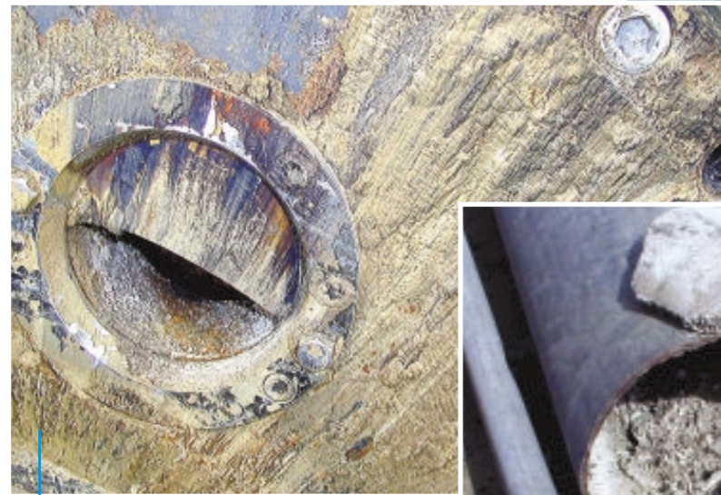
Deposition on the end wall of a centrifuge
